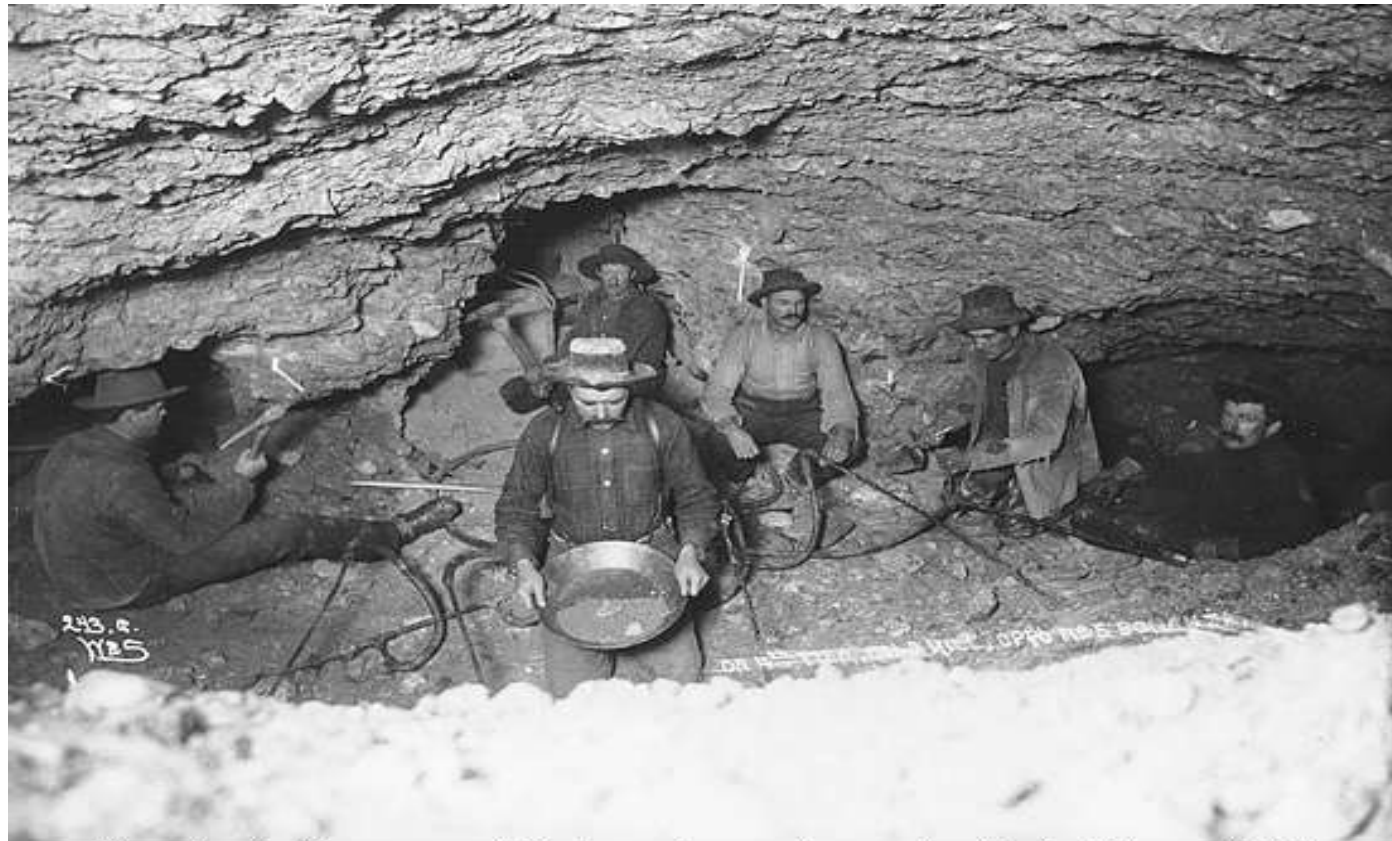
Miners thawing frozen ground with steam in an underground gold mine lit by candlelight, Gold Hill, Yukon Territory, ca. 1898
